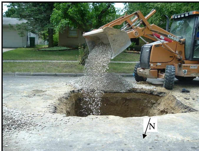
Figure 57 - Front-end loader operating on the southwest side of the trench
