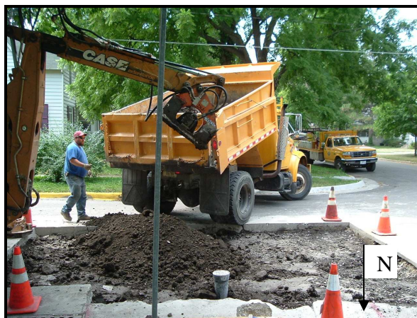
Figure 59 --Soil removed from the trench being placed back into the trench by a truck located on the south side of the trench, and a backhoe operating on the east edge of the pavement for Trench E
