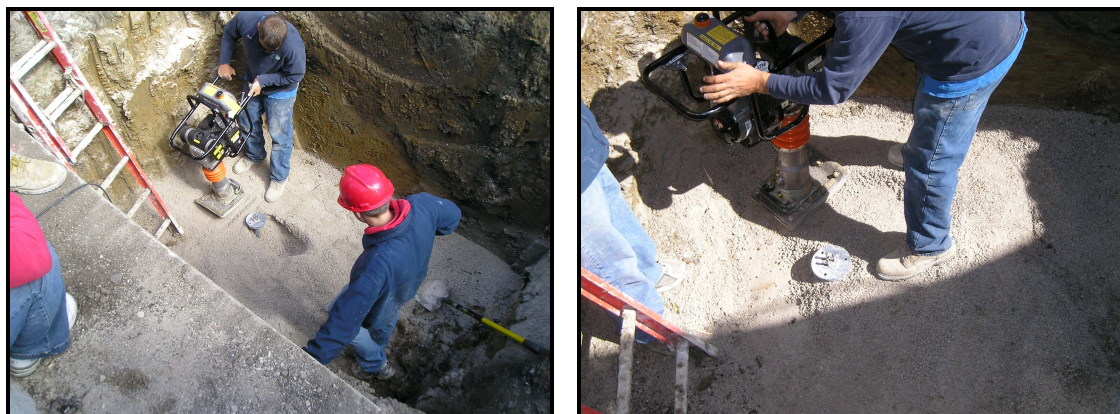
Figure 183 – a) Extensometer being moved back to vertical alignment and b) final compaction around the extensometer after being re-aligned with vertical
