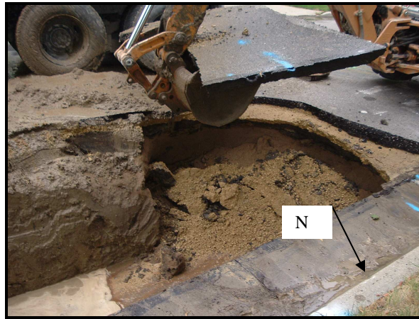
Figure 44 -- Backhoe operating on southeast edge of Trench A
