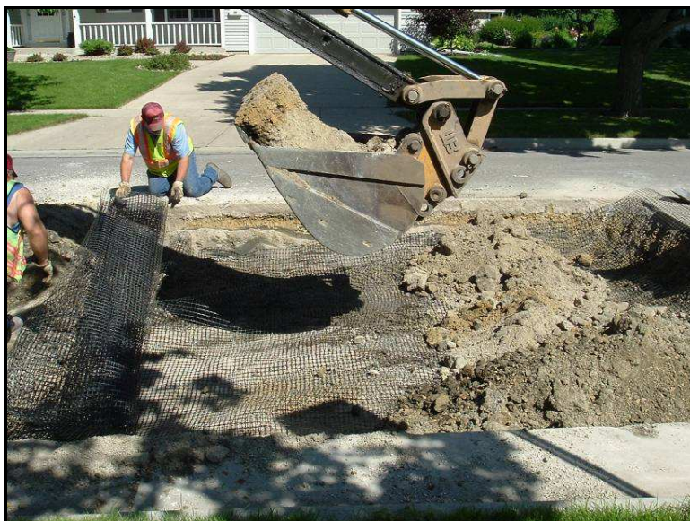
Figure 54 -- Geogrid being placed in Trench C
