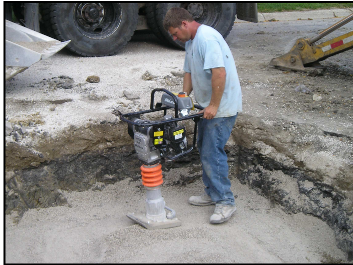
Figure 175 -- Impact rammer used to compact the backfill in Trench 1
