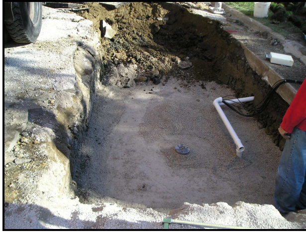
Figure 185 – The excavation of the T-section being constructed for Trench 3
