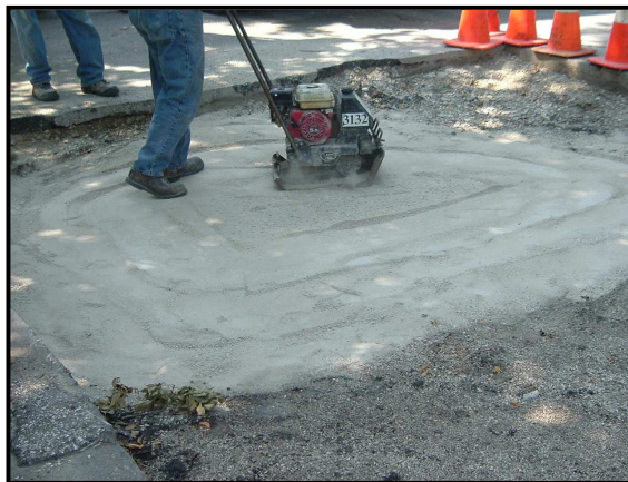
Figure 50 -- Small vibratory compactor used to compact the backfill
