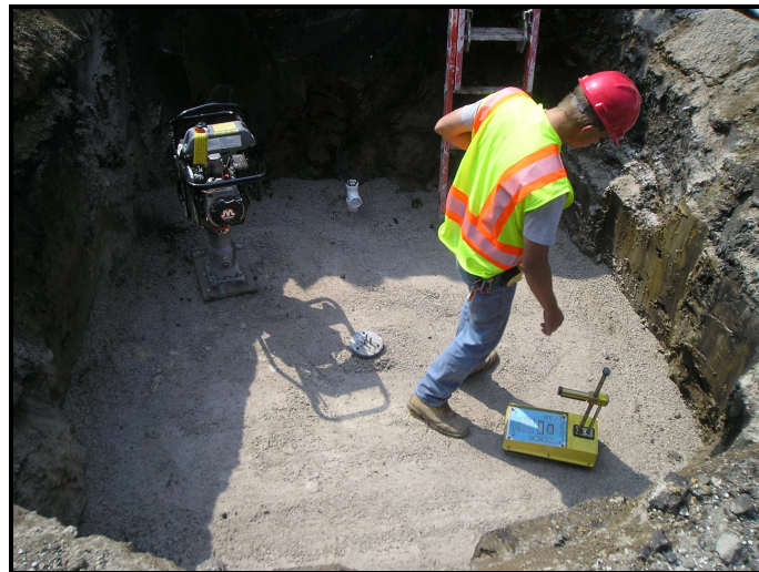
Figure 176 -- Nuclear density gauge used in Trench 1
