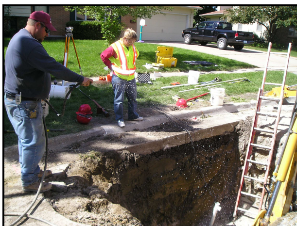
Figure 183 – a) Extensometer being moved back to vertical alignment and b) final compaction around the extensometer after being re-aligned with vertical
